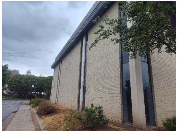
Photo 4: View of the western side of the Site building.
