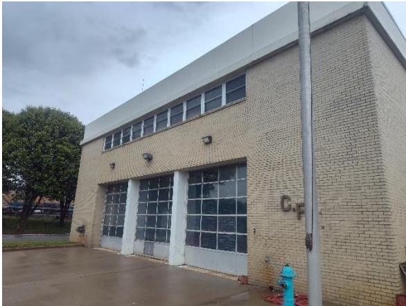
Photo 1: View of the western side of the Site building.
