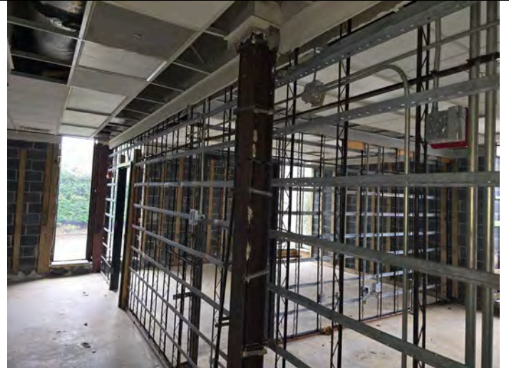
Photo 2 – Red metal I-beams throughout the 1 st & 2 nd floor - LBP
