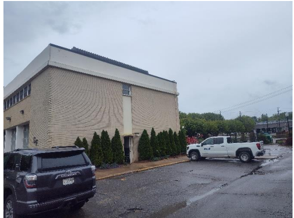
Photo 2: View of the southern side of the Site building.
