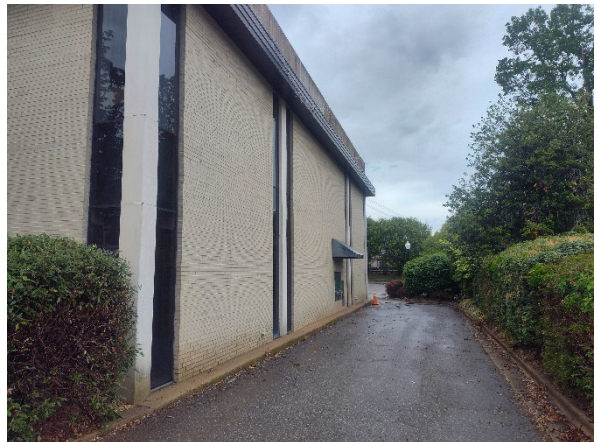
Photo 2: View of the eastern side of the Site building.
