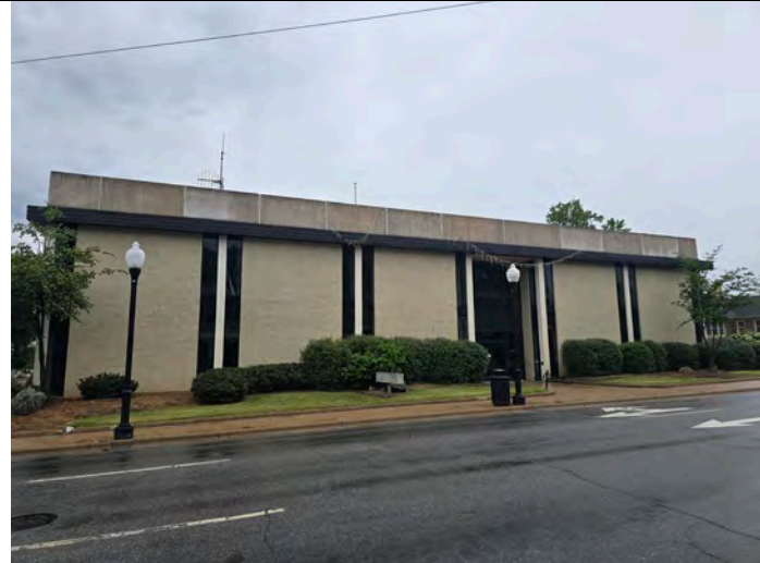
Photo 1 – The former Town Hall located at 58 Park Street, Canton, NC 28716
