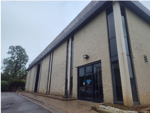
Photo 1: View of the northern side of the Site building.
