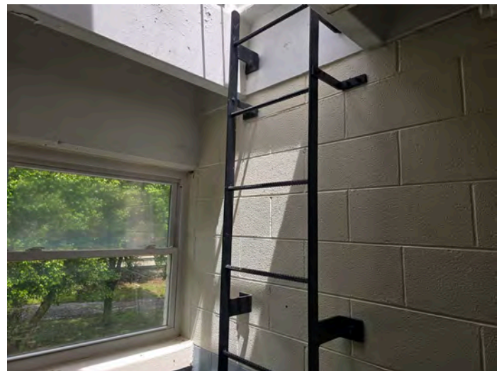
Photo 6 – Black metal roof access ladder in one of the stairways - LBP
