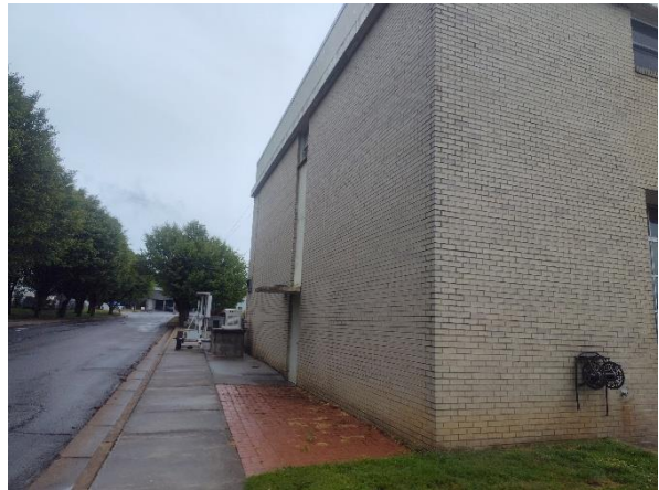
Photo 4: View of the northern side of the Site building.
