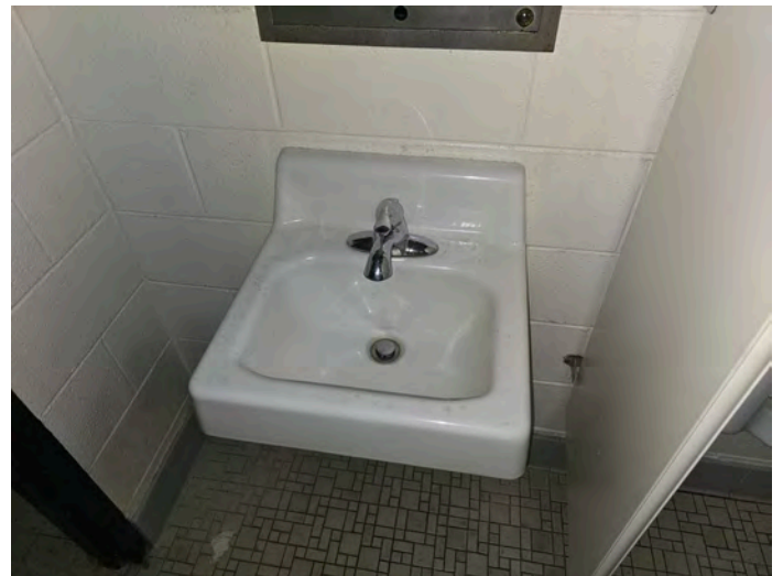
Photo 4 – Typical view of a white metal sink in the bathrooms
