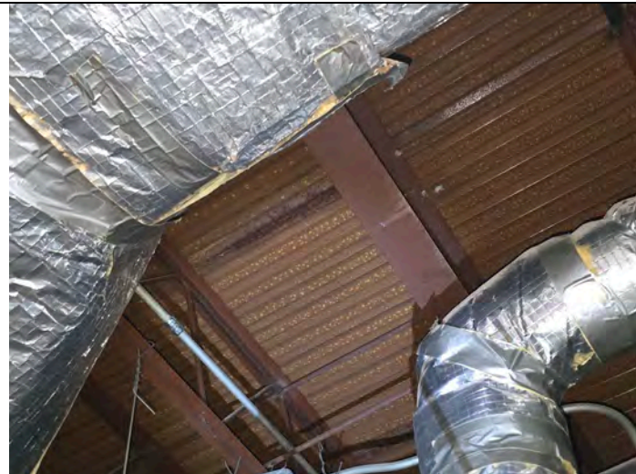
Photo 3 – Red metal I-beams throughout the 1 st & 2 nd floor - LBP
