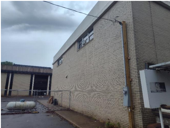
Photo 3: View of the eastern side of the Site building.
