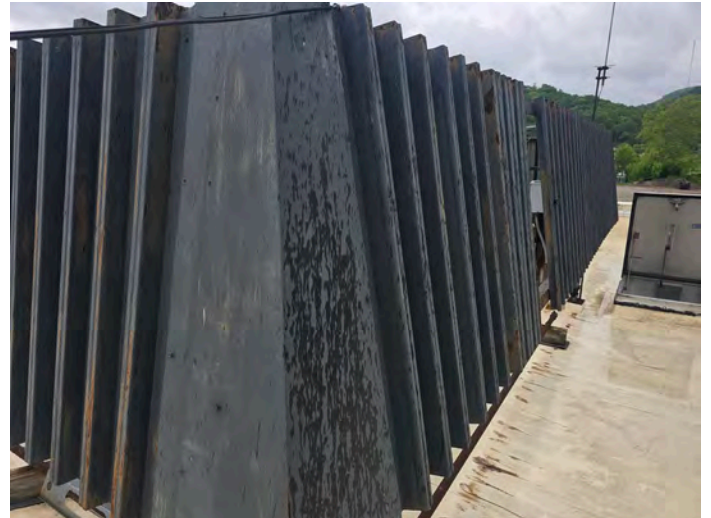
Photo 2 – Green metal wind barrier on the roof – LBP
