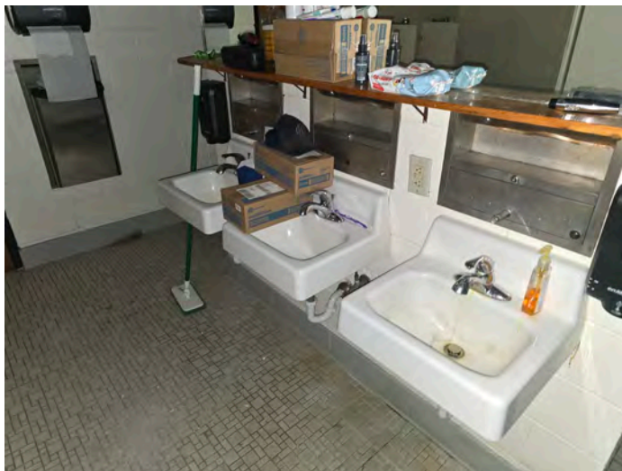
Photo 5 – Typical view of a white metal sink in the bathrooms
