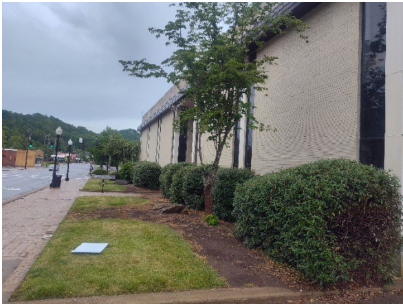
Photo 3: View of the southern side of the Site building.
