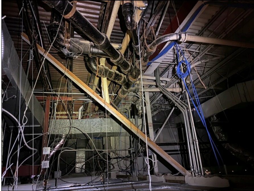
5 - View above the second floor drop ceiling.
