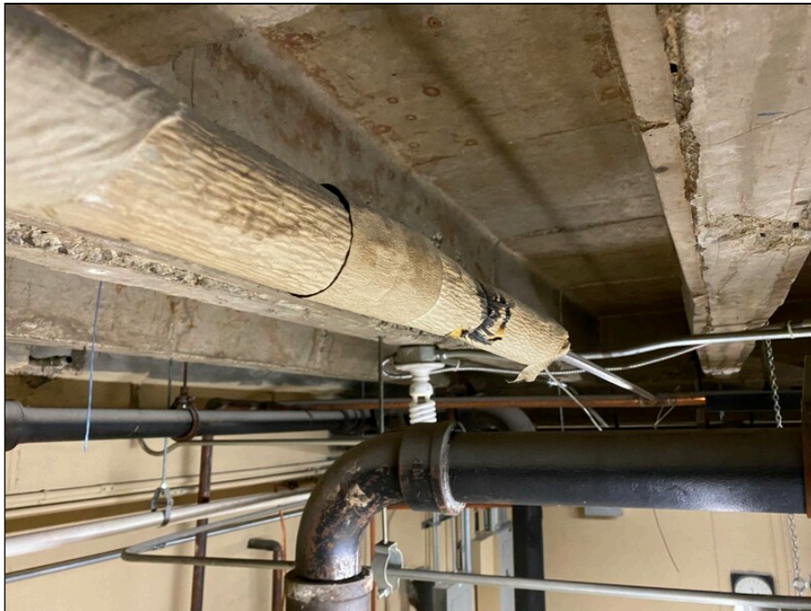
8 - View of fiberglass piping, with ACM white mudded fittings.
