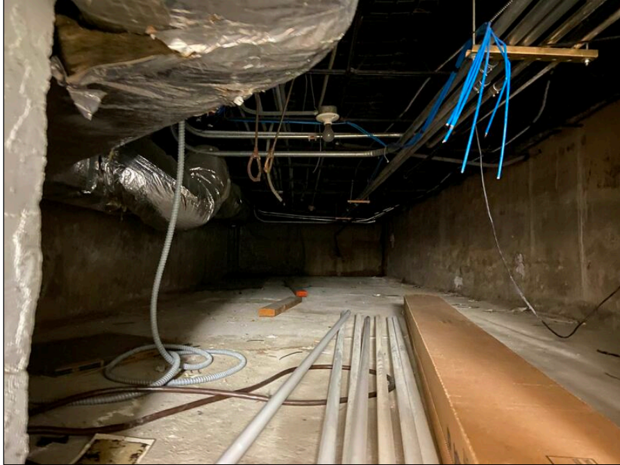
5 - View of crawlspace
