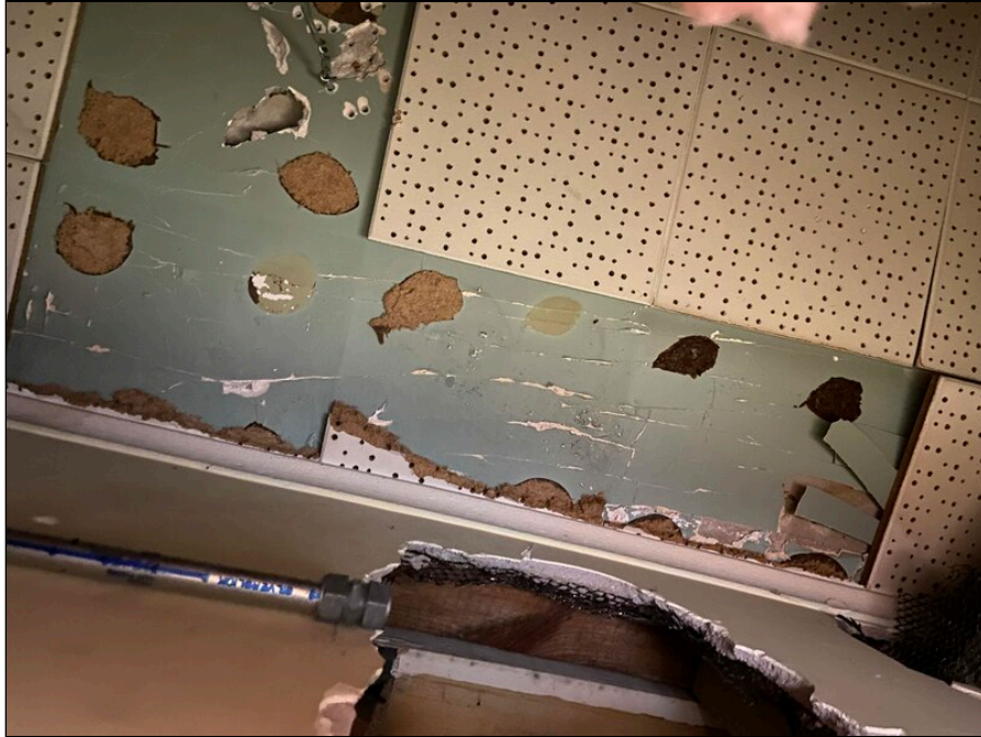
7 - View of original ceiling tiles above drop-down ceiling
