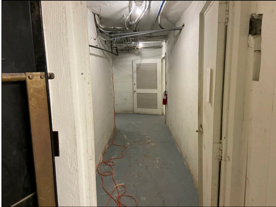
3 - View of basement
