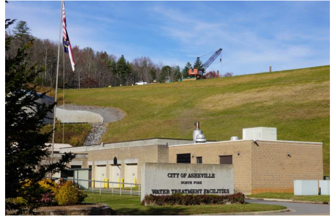
FEMA, U.S. Army Corps of Engineers and the Environmental Protection Agency worked alongside the city of Asheville to restore its water service after repairs and water treatment at the North Fork Reservoir after Tropical Storm Helene caused severe damage to the facility.
